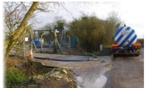
Sewage Treatment Plant in Brize Norton. Pumping for weeks on end!
