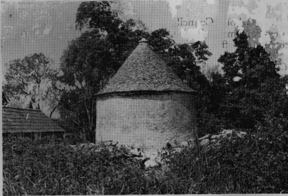
The Dove Cote, Grange Farm
