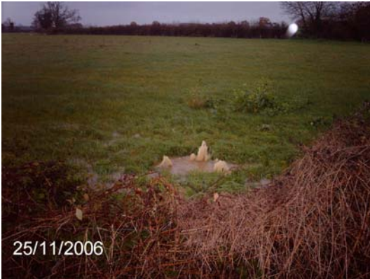
Sewage spewing into the field.
